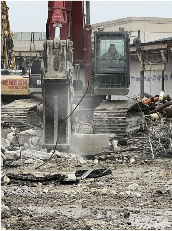
Photo-3: Close up of concrete being pulverized to separate rebar.
